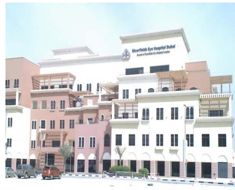
Moorfields Hospital in Health Care City, Dubai *1 unit of 40kVA
