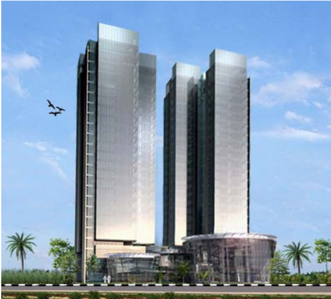
Novotel & Ibis towers - AD
