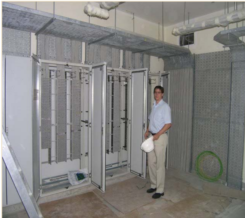
Dubai Airport Free Zone – Phase IV MDF Room
