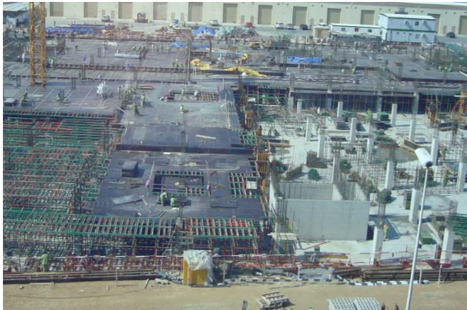
Dubai Airport Free Zone Phase VII – Dubai
