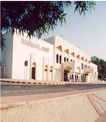
FUJAIRAH INTERNATIONAL AIRPORT *1 unit of 40kVA *2 units of 20kVA *1 unit of 10kVA
